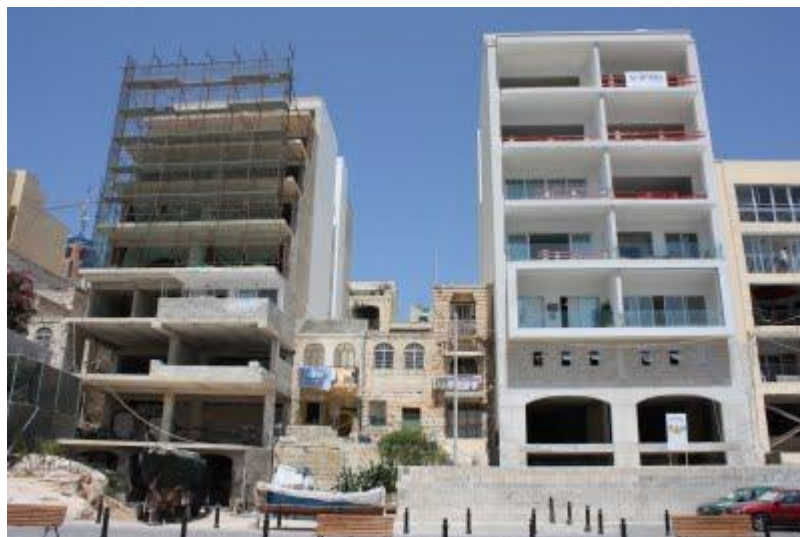
Figure 2: Modern architecture, characterised by high rise buildings and pre-fabricated concrete
